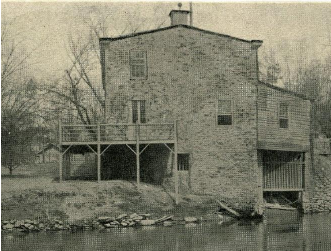
1906 Porch added with door, pre-Creek Wall
